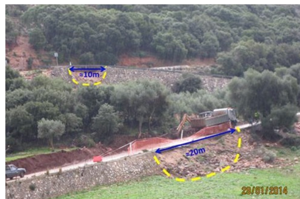
Picture 11. Typical failure types of stone retaining walls recorded after the Lefkas, 2015 (left) and Cephalonia, 2014 (right) earthquakes
