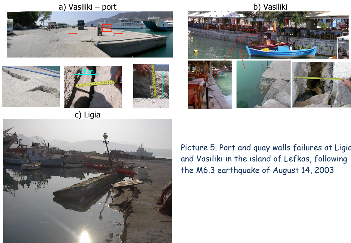
Picture 4. Earthquake-induced failures at the port of Lefkas, following the M6.3 earthquake of August 14, 2003.
