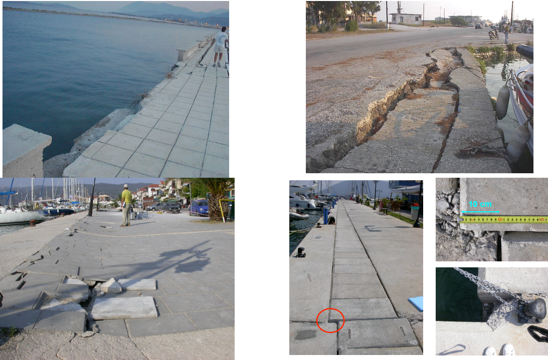
Picture 4. Earthquake-induced failures at the port of Lefkas, following the M6.3 earthquake of August 14, 2003.
