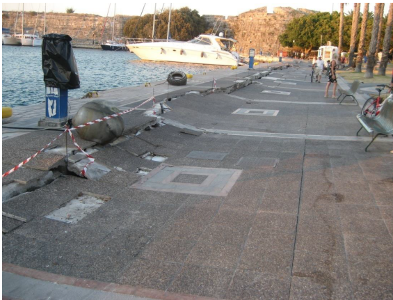
Picture 6. Earthquake-induced failures at the port of Kos, after the strong M6.7 earthquake.
