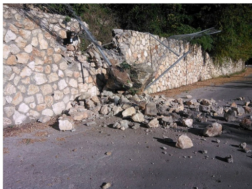
Picture 11. Typical failure types of stone retaining walls recorded after the Lefkas, 2015 (left) and Cephalonia, 2014 (right) earthquakes
